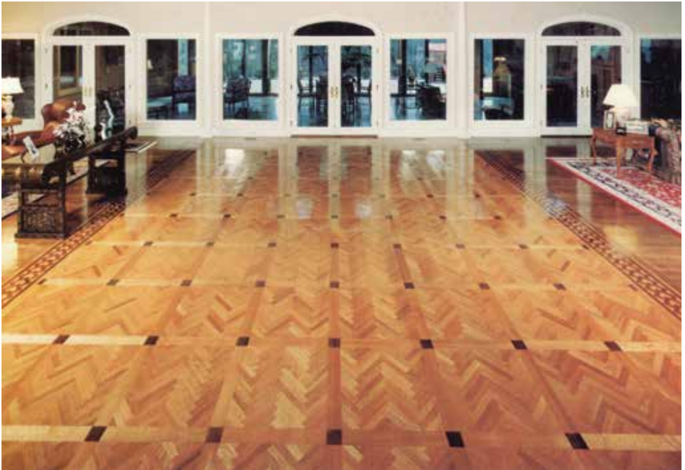
This residential homeowner originally had no clear idea as to what they wanted for their in-home corporate entertainment space. The JJ Hardwood Floors team came up with this custom on-site design for the ballroom. Each box is individually built with 2 ¼ rift and quarter Red Oak, 4” by 4” walnut blocks in each corner of all the boxes with a 4” rift and quarter band around each herringbone box. The border detail around the perimeter of the room is a laser cut walnut border with diamond inlays. The sanding process involved took three days just to stain the herringbone field and three more days to finish with oil-base polyurethane.
