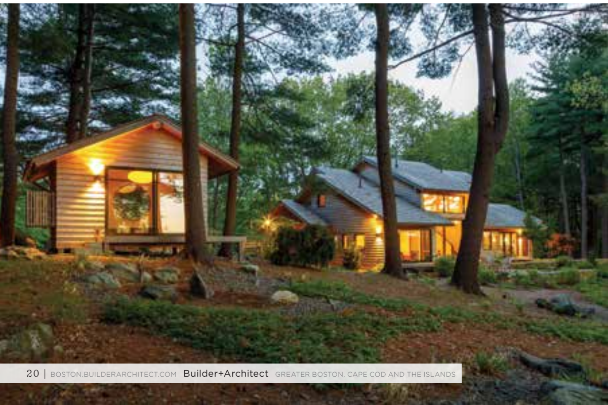
Built for the owner to have their traditional tea, the adjacent teahouse is 13 feet by 9 feet and faces the Merrimack River. The corners of the teahouse represent Respect, Purity, Harmony and Tranquility.
